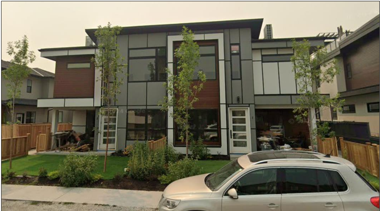
Figure 2 – Front Façade at 867 Morrison Avenue.
